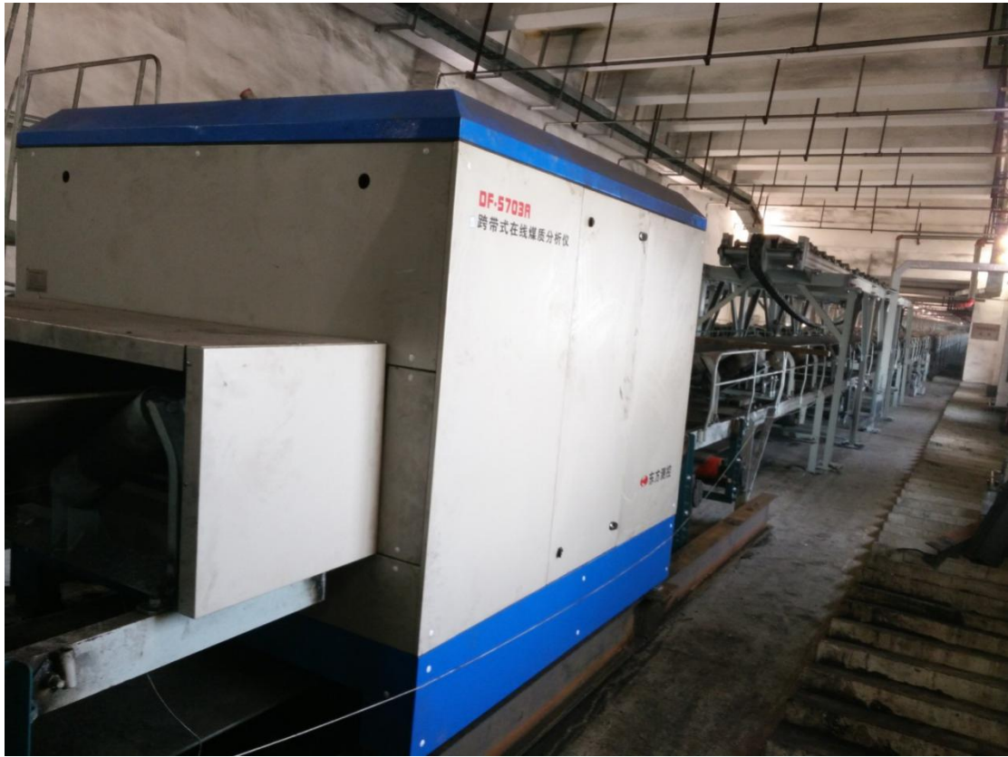
Fushun Ore Zhongji Thermal Power Co., Ltd.
